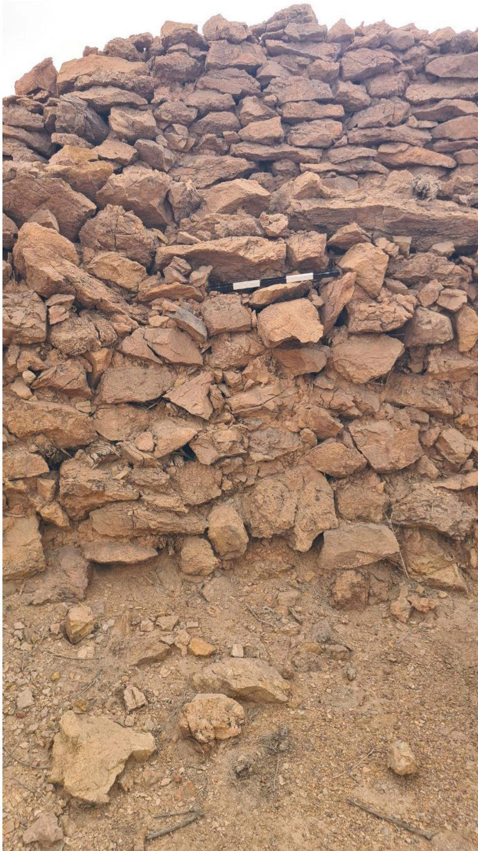
Fig. 35: The walls of F42 from the inside. The location of the wood sample we took is marked by the yardstick
